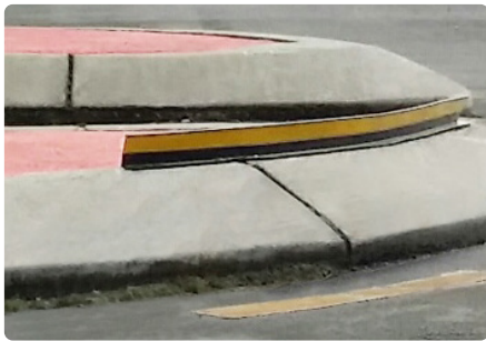
As installed in Rangiora, Canterbury
