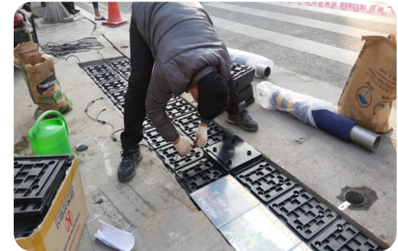
Fix top tactile plates into position and silicone
