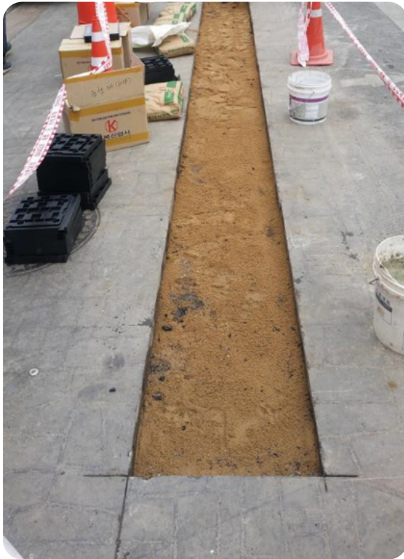
Cut out pavement for LED tactiles
