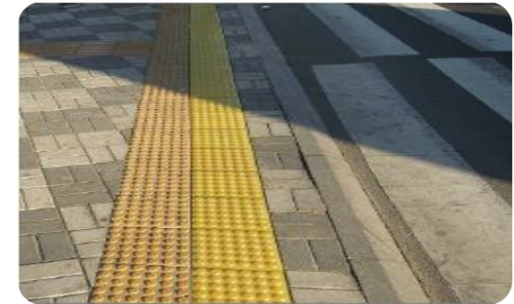
Fix top tactile plates into position and silicone
