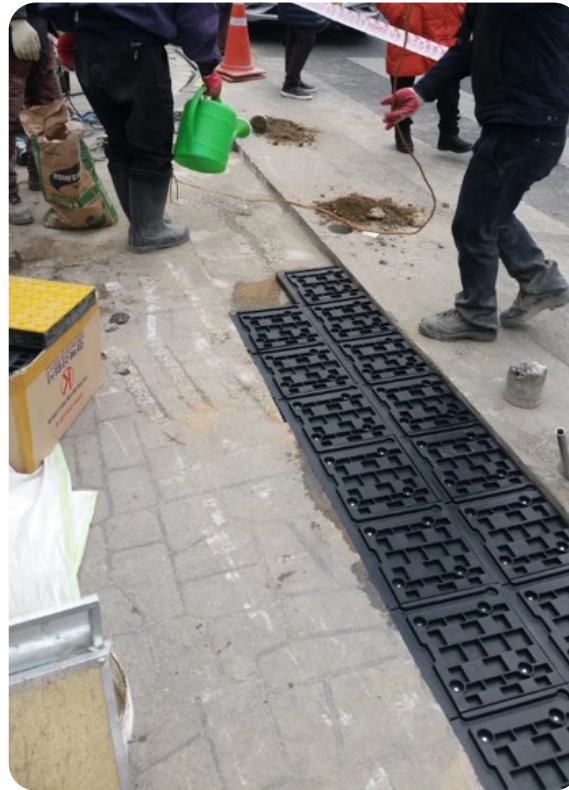
Cement and fix base plate into ground
