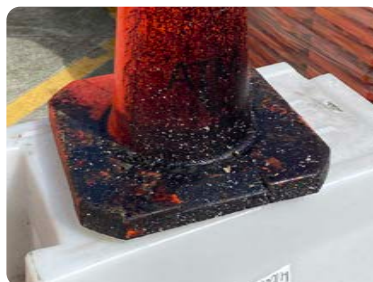
Excessive Bitumen
