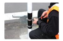
Note: At this stage, do not overly tighten brackets, as some adjustment made be required for the School Patrol Arm to lift up into the Top Cover. NEVER CLAMP DIRECTLY ONTO THE REFLECTIVE BANDS.
