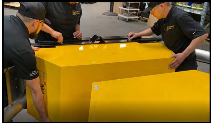
2. Secure Module C with washers and Button head bolts. Use grease on all bolts and tighten to a minimum of 20 ft-lbs.
