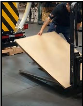
5. Place a piece of cardboard on the forklift to prevent damage to the TMA diaphragm.
