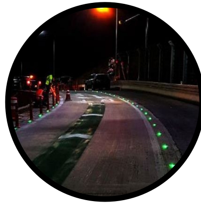
Solar Powered Stud Lights Installation
